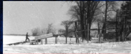
Every February, with hired help, ice was harvested from the bay. Blocks were sawn from the ice and taken up the slides into the ice house as shown. Sawdust from local lumber mills was used to cover the top and sides of the ice. This ice was then delivered to cottages and some businesses throughout the summer.
