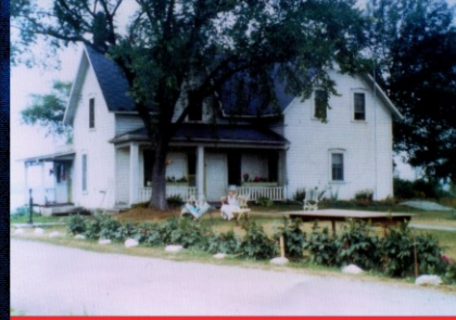
The Atkins family home, circa 1940. At the left is a water pump used to supply the family's drinking water. The concrete slab it stood on, located to the left of this sign, is all that remains today of the Atkins farm complex.
